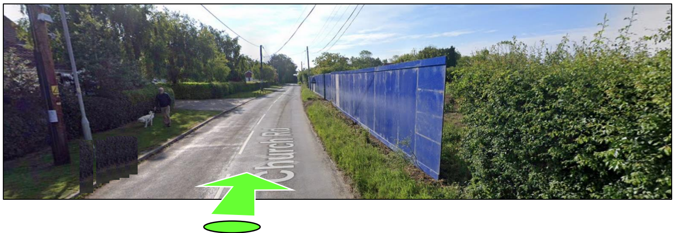
figure 2: The site's Church Road frontage [blue hoarding] [green dot and arrow refer to figure 1 viewpoint]
